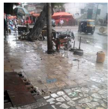
Shards of tiles on the pavement of the old town of Hamarweyne. This system is catching on in Mogadishu on sidewalks and the pedestrian places is a major threat to the safety of pedestrians because they are very slippery.
