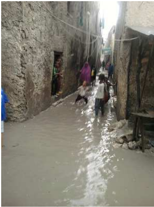
After a heavy rain in an alley that leads to the area of the mosque Jaama'a.
